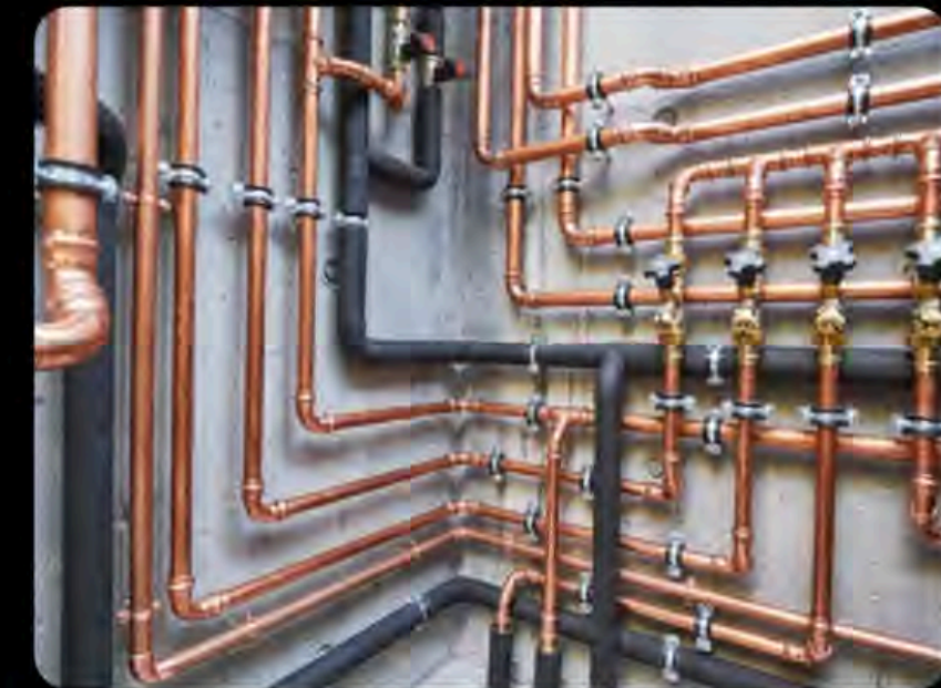
Plumbing perfection thanks to trigonometry
